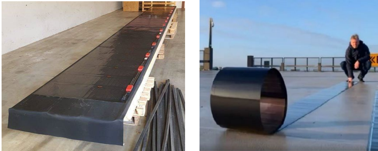
Figure 6: Left: In 2020, for the 9.2 meter long laminate in the STAL-project, manual stitching was still needed. Right: In 2022, a 10 meter long laminate has been produced without stitching.
