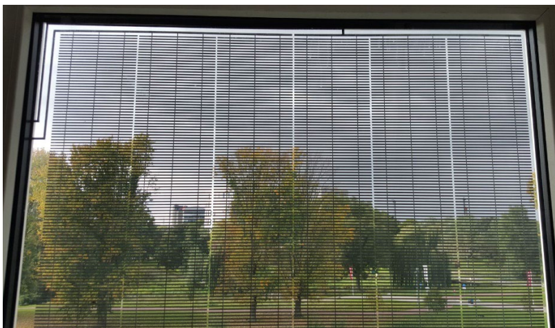
Figure 19: IGU with transparency achieved by using small c-Si PV cell-strips. © Pilkington Sunplus™ BIPV [20]
