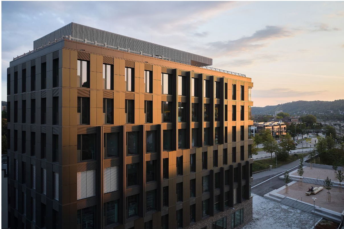
Figure 21: Avancis Skala at Westspitze, © Avancis, Albrecht Voss. Source: https://www.skalafacade.com/en/
