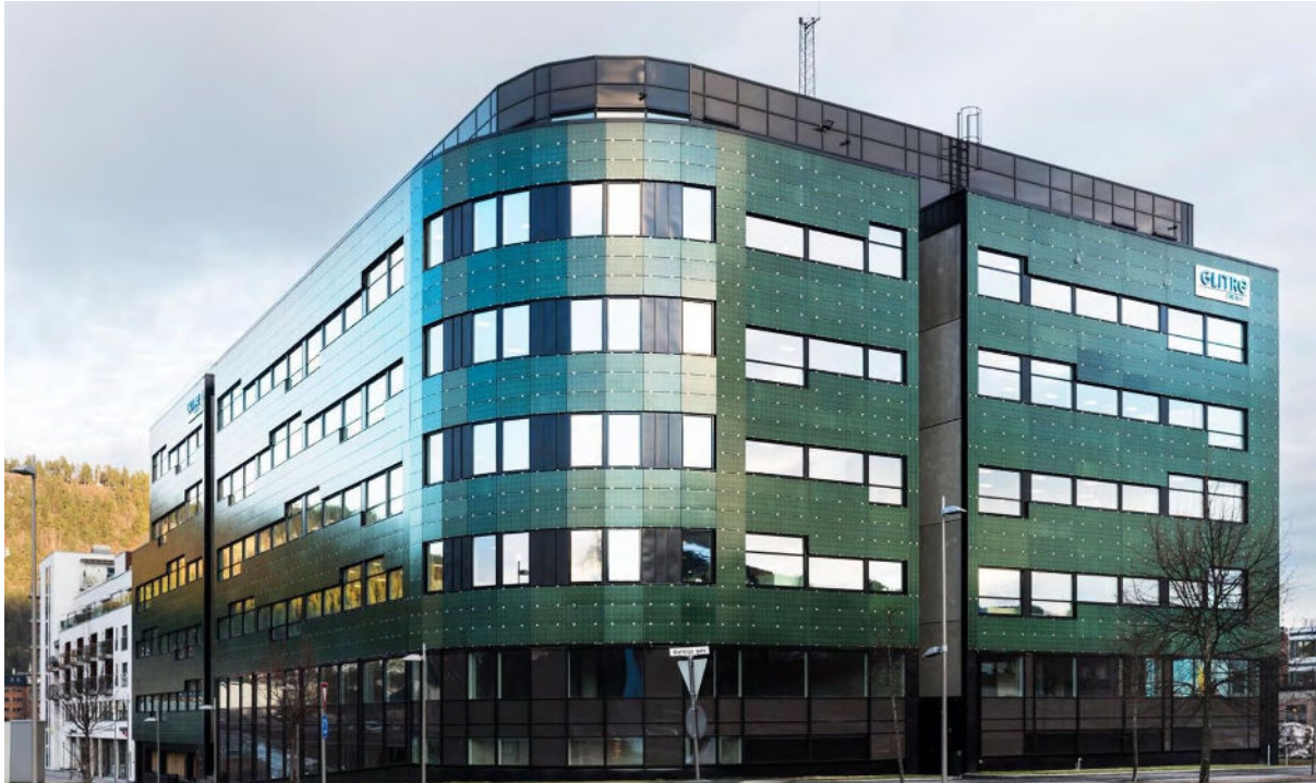
Figure 31: Solsmaragden Offices, Drammen (NO), © Enova. Source: https://iea-pvps.org/wp-content/uploads/2021/03/IEA-PVPS-Task-15-An-international-collection-of-BIPV-projects-compr.pdf
