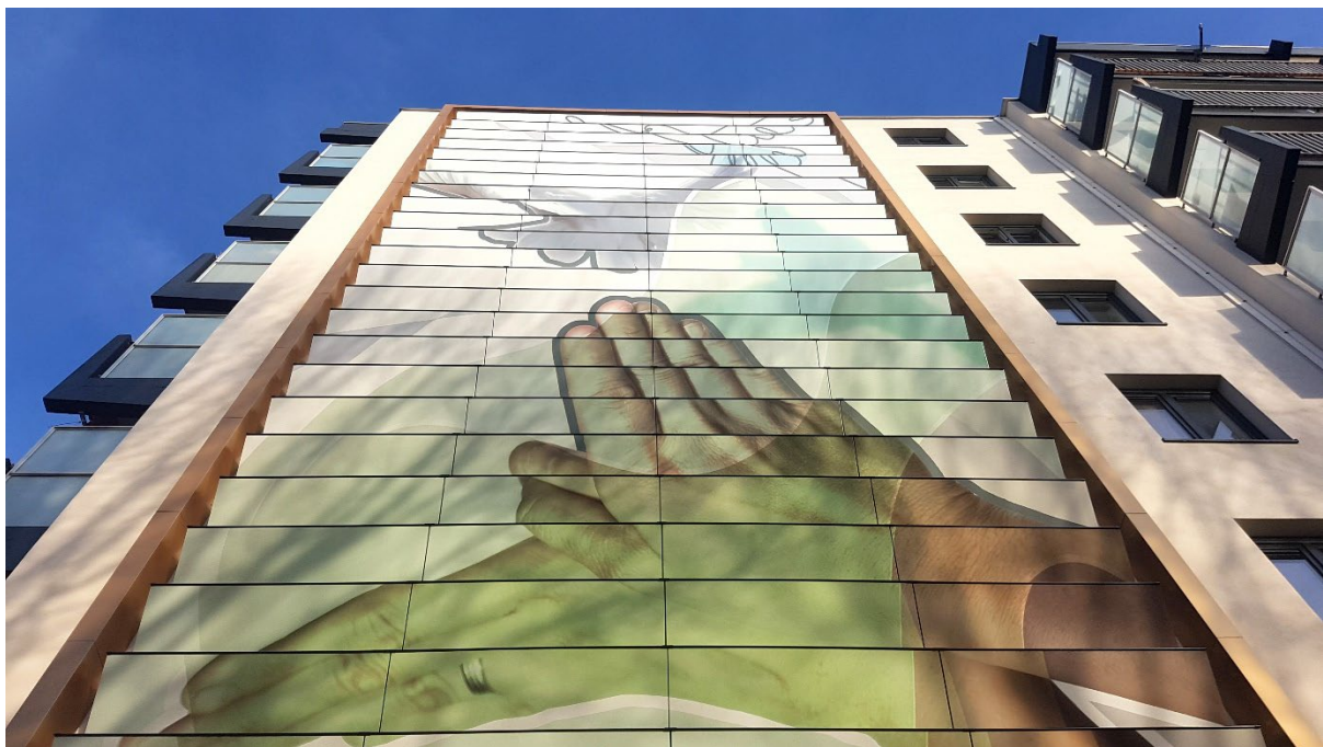
Figure 11: ZigZag solar has a regular product that is already custom-made with respect to the color and patterns on the downward facing parts of the façade. The PV-panels are integrated in the upward facing part and therefore invisible from ground level.
